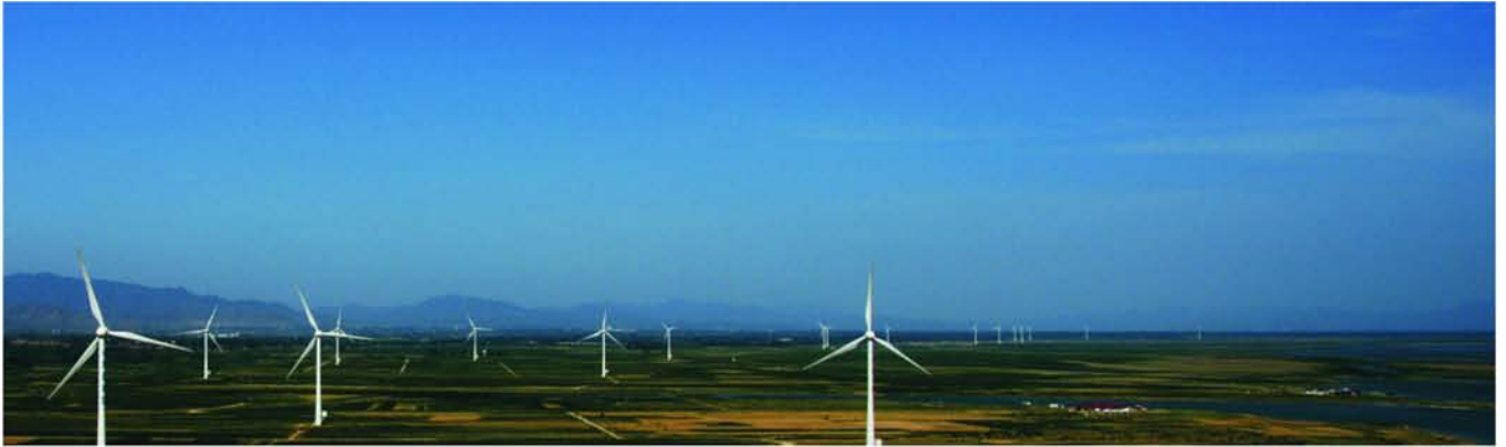
The Guanting Wind Farm
